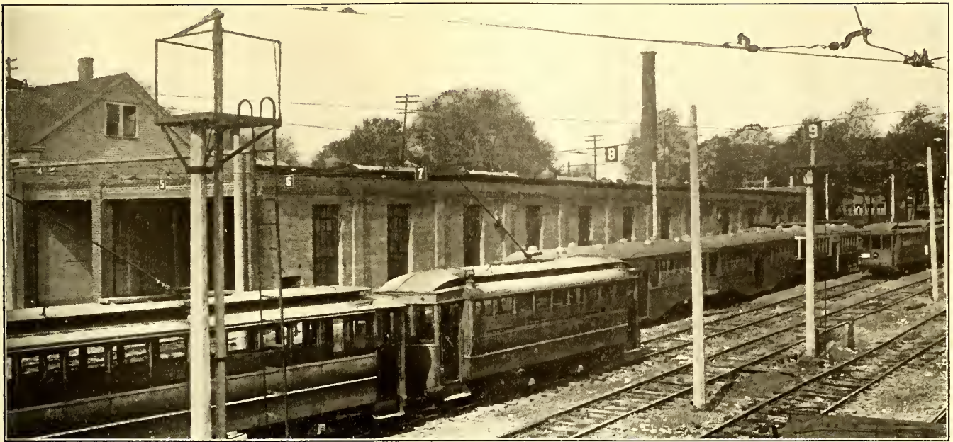
ROCHESTER CAR-YARD IMPROVEMENTS—VIEW IN YARD WITH MONITOR NOZZLE SPRINKLER POLE IN FOREGROUND
